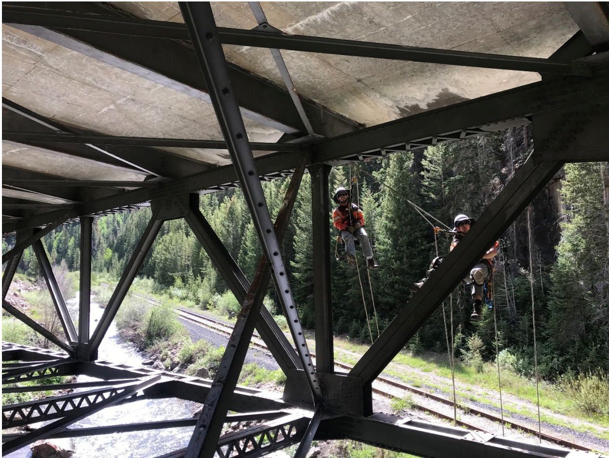
Figure 6-12: Bridge Inspection with Rope Access. Source: Engineering Operations, CDOT
