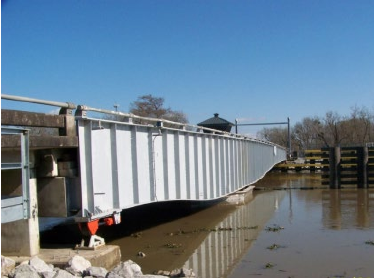
Figure 6-6: Steel Plate Girder Swing Span
