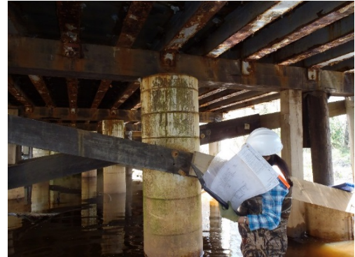
Figure 8-1: “Field” Review of Bridge Inspection
