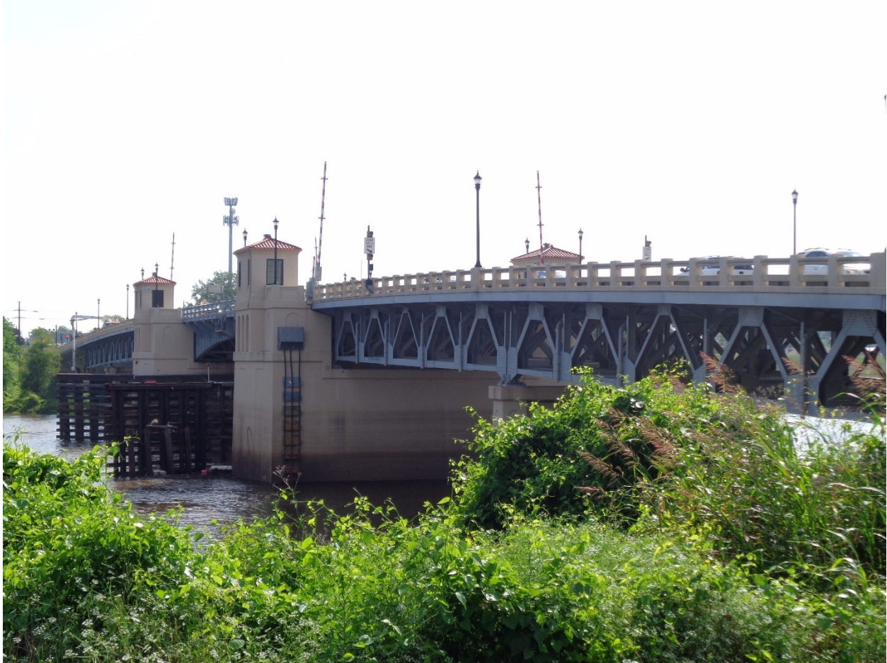
Figure 6-8: Steel Truss Bascule Span
