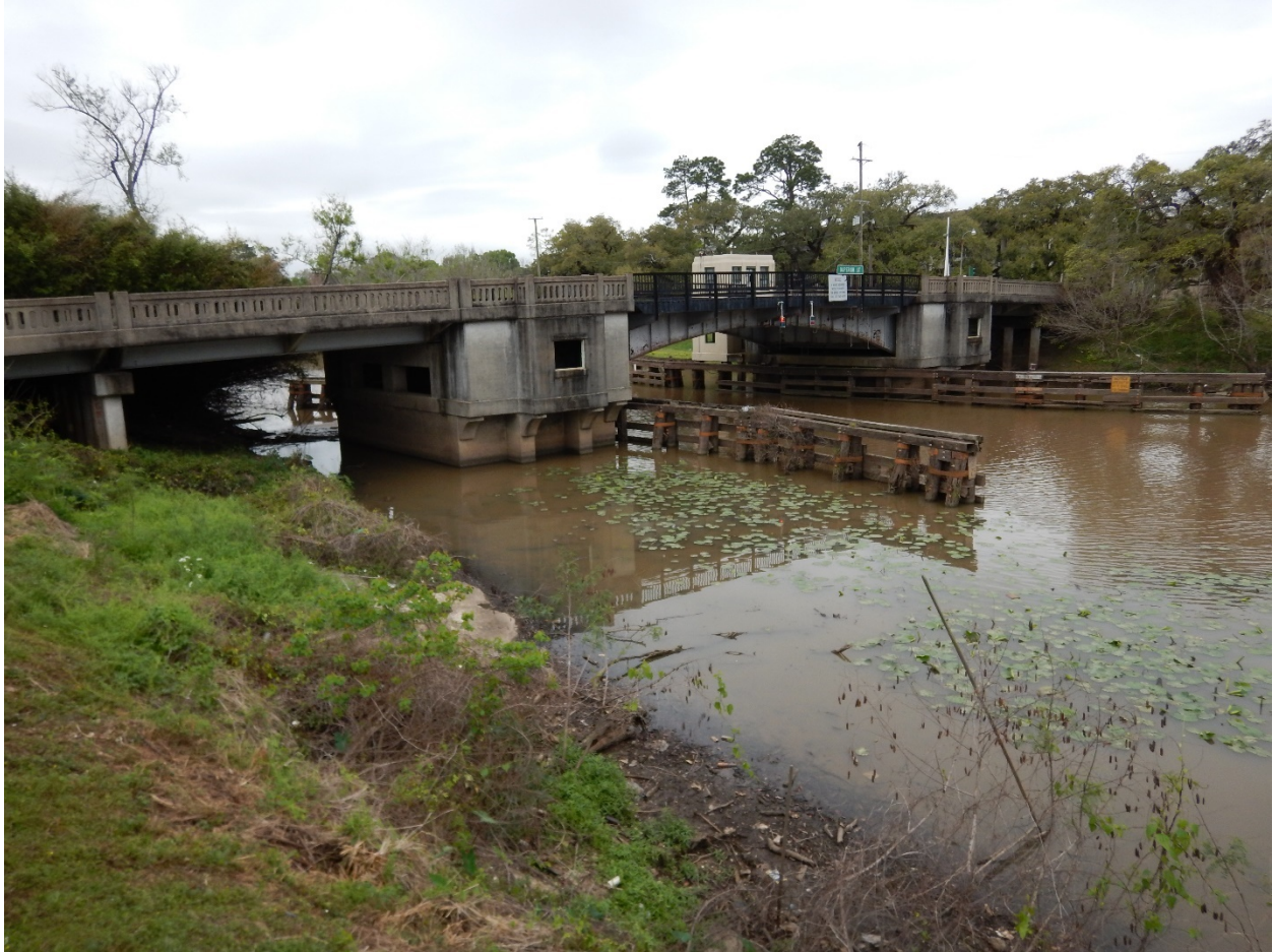
Figure 6-9: Steel Plate Girder Bascule Span. Source: Moffatt & Nichol, LADOTD
