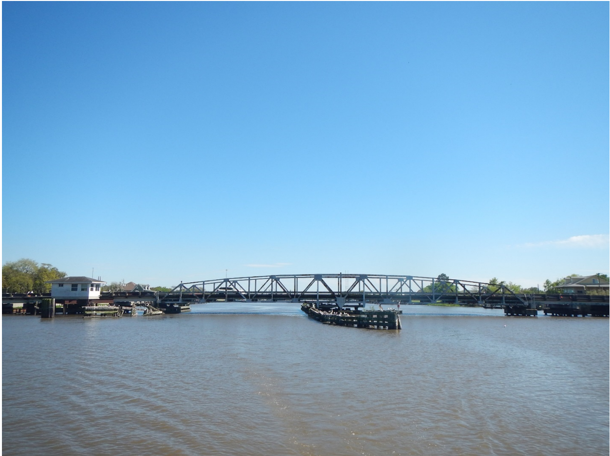
Figure 6-5: Steel Low Truss Swing Span
