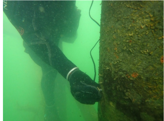
Figure 5-4: UT on Steel Pile. Source: Engineering Operations
