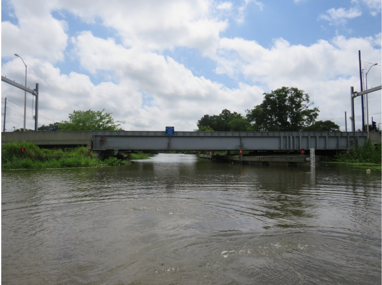
Figure 6-7: Steel I-Beam Swing Span
